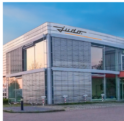
JUDO Hertmannsweiler: New production facility for industrial and building technology
